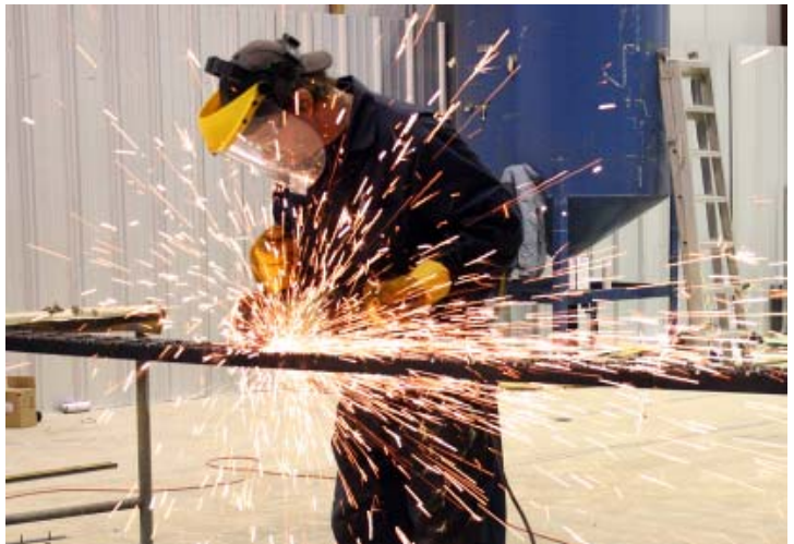
Welder cutting Floor Grates at Enviro-Pads
